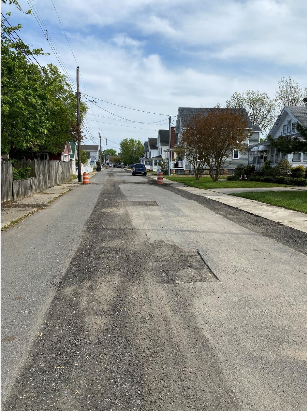
Cropper Street Storm Drain Installation Complete on 4/25
